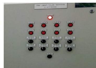
Gambar 12 Interface Relay Panel (IRP)
