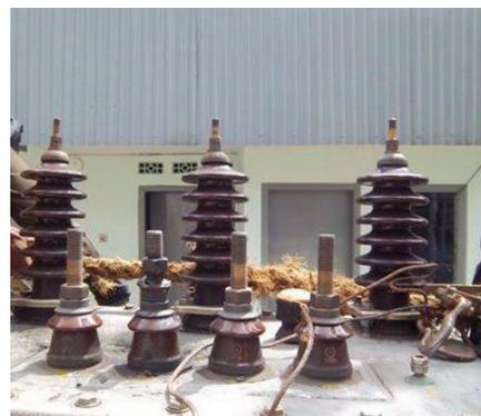
Gambar 4. Bushing Transformator
