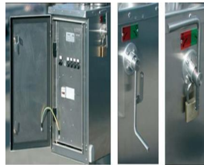
Gambar 10. Drive Mechanism Manual
