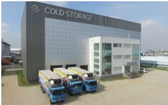
Gambar 2. 1 Cold Storage Statis (Sumber: Foto KKP)
